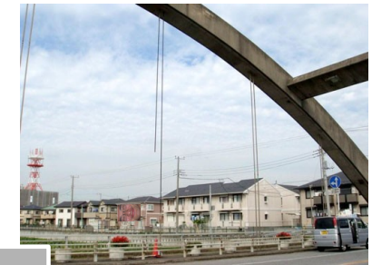
吊材の破断 (君津新橋)
